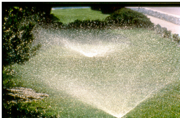
Figure 1. Fixed spray heads traditionally used in landscape irrigation produce a static spray over their arc of coverage.
