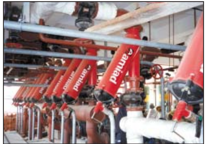
"Siemens Power Station" - China. Semi automatic filtration for the cooling water system, 300 micron.
