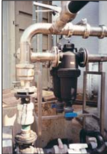
Filtration of process water in a detergent manufacturing plant
