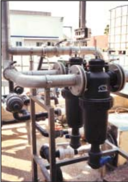
Filtration of process water in a detergent manufacturing plant
