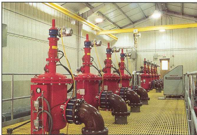
Zebra mussel protection at fish hatchery. Vermont, USA.
