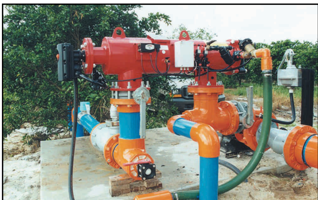
Sprinkle irrigation of citrus grove. Florida, USA
