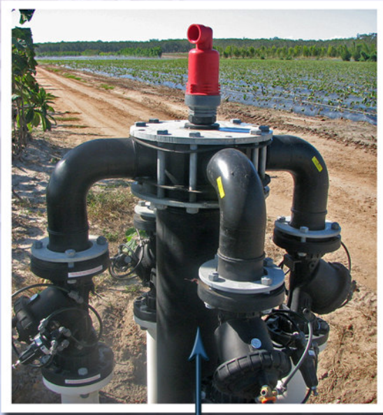
Flow Dividers allow 360° rotation as well as bolt-on upgrades
