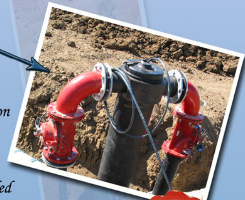
Large bore socket to flange tees using Maxi Stub to allow valve opening without the need for spacers
