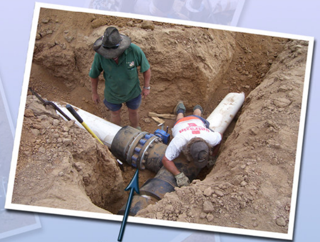
Large bore socket to flange tees using Maxi Stub to allow valve opening without the need for spacers
